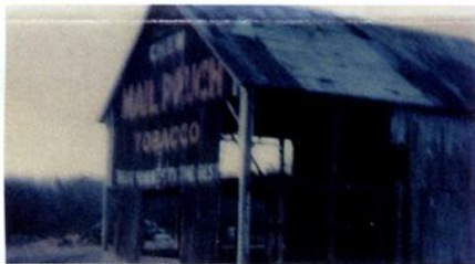
OUR FIRST WAREHOUSE
